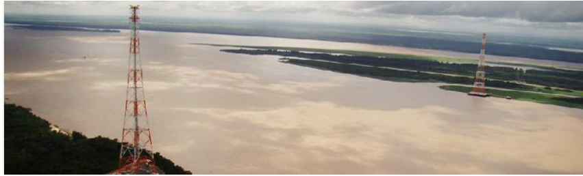
Fig. 12 Jurupari crossing looking eastwards (downstream) (Courtesy of Isolux-Corsán)
