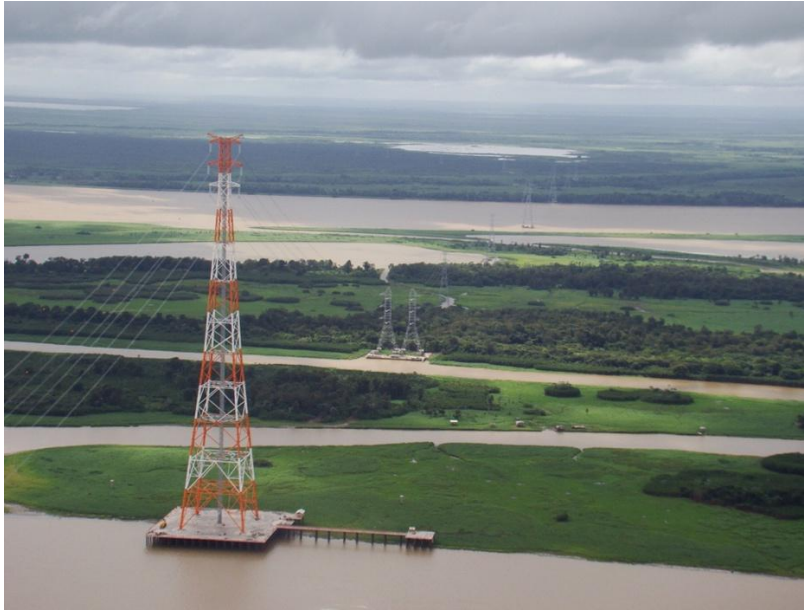
Fig. 14 Jurupari crossing looking southwards. (Courtesy of Isolux-Corsán)
